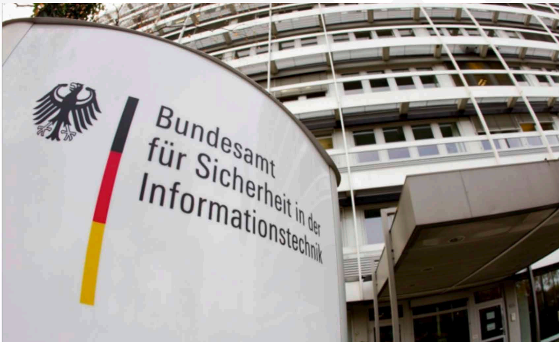
Figure 2: Building of the German Federal Office for Information Security in Bonn, Germany
